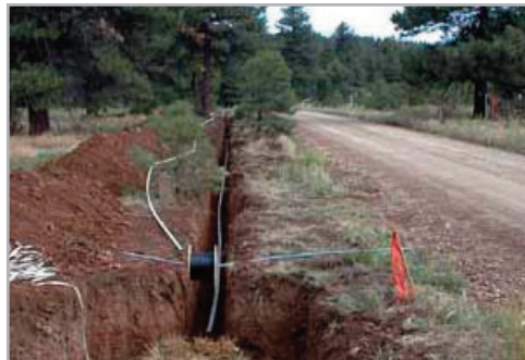
Electric and phone trench
