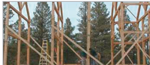
Placing bent 3
