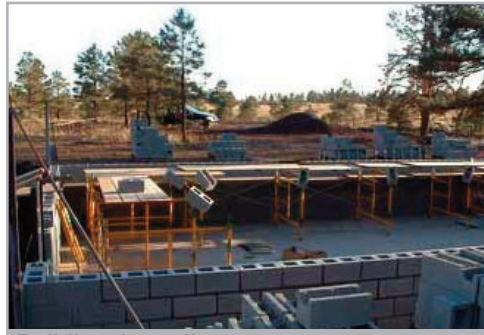
Building the walls
