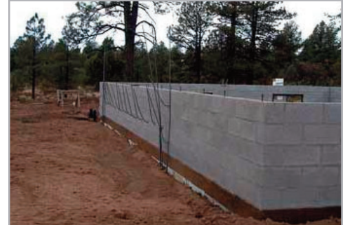
Back filled—garage side
