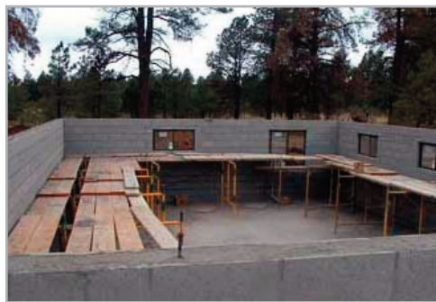
Completed basement / interior
