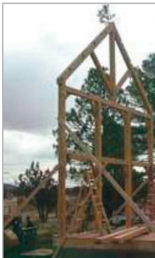
Bent 1 (front wall)
