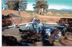
Radiant heat work
