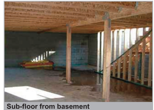
Sub-floor from basement
