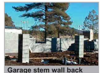
Garage stem wall back
