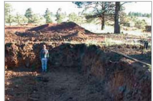
Chris, standing in the foundation hole.
