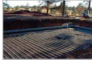
Final radiant tube layout
